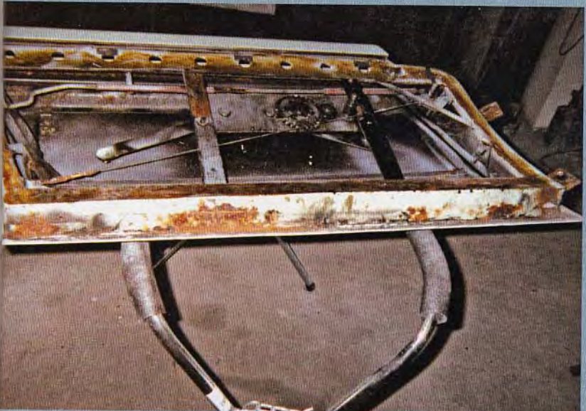
What looks like rust is adhesive from weatherstripping added later. Diagonal wire holds door square, in tension. New glass was cut locally
